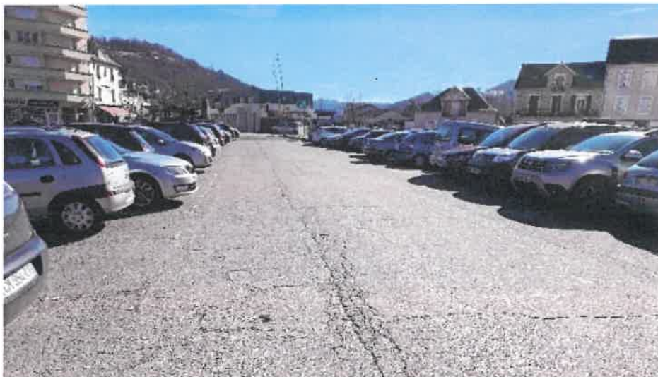
Figure 4 : Parking du CCS
